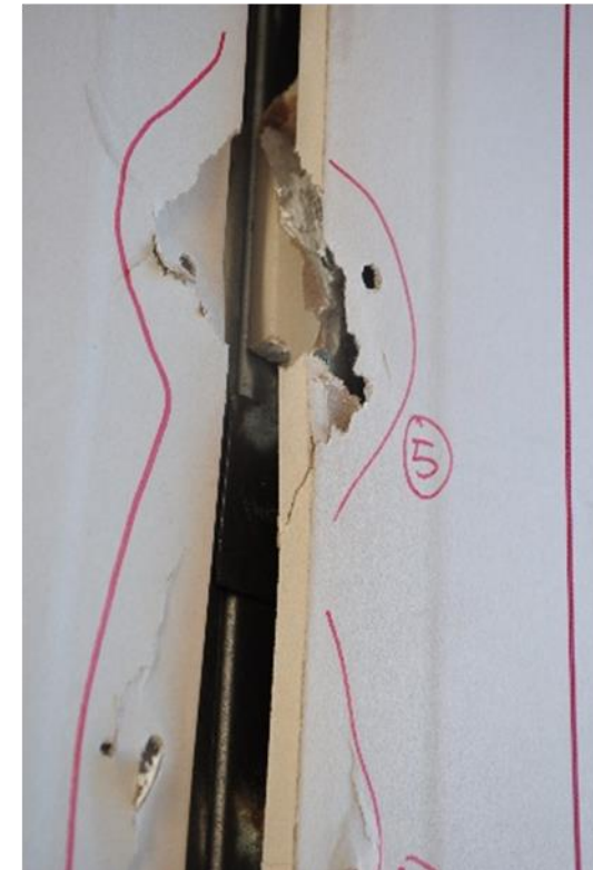
Extensive damage to Gypsum boards
