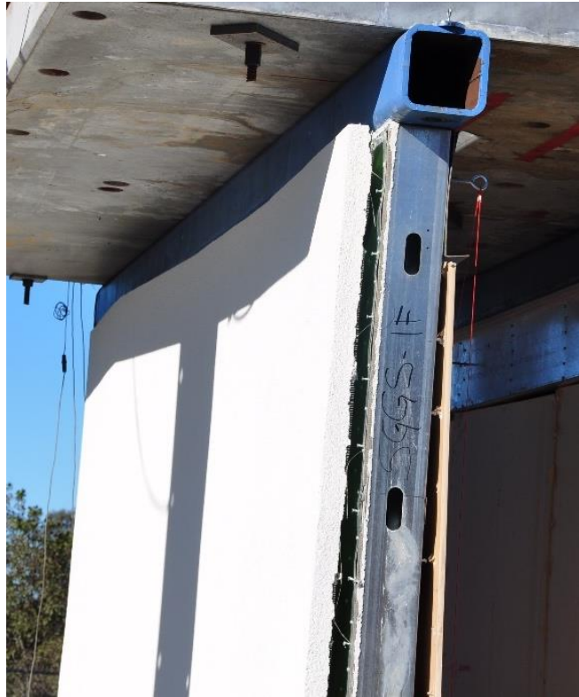
Separation of finish layer from steel sheet with screw pull through
