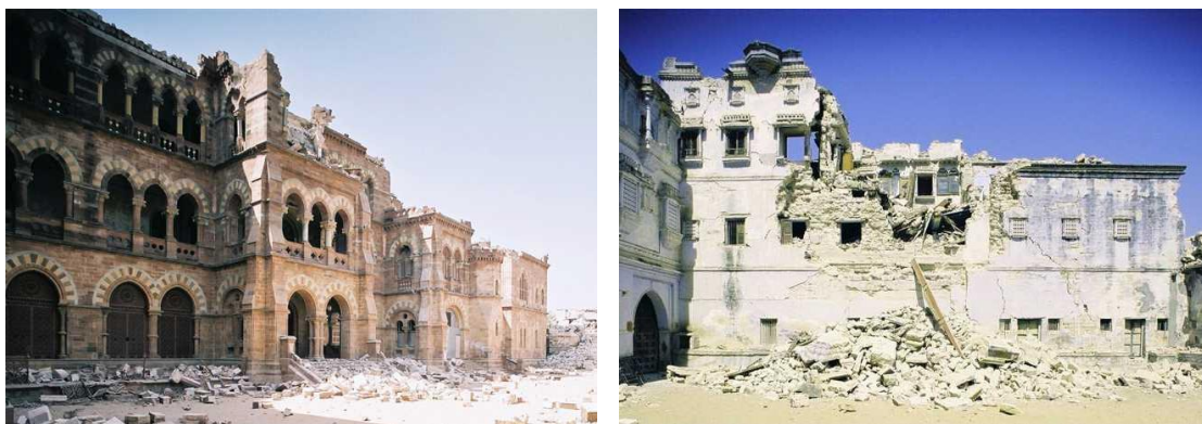
Figure 1.4. Damage to heritage structures in Kutch region of Gujrat due to M7.7 Bhuj earthquake of 26 th January, 2001 (UNESCO Report 2001)
